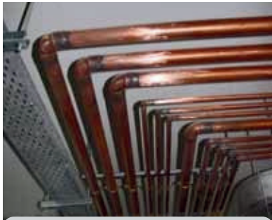
Piped Medical Gas Systems
